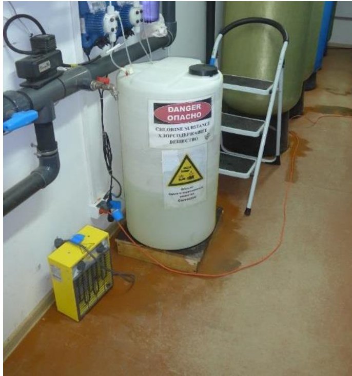
Photo 23 – Drum of hypochlorite without secondary containment
