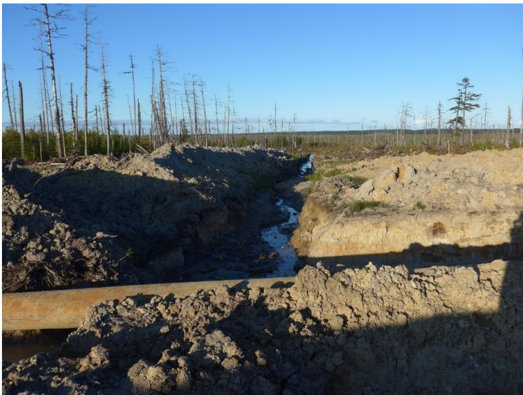
Photo 31 – Ditch adjacent to stormwater retention pit in the north of the OPF-C site
