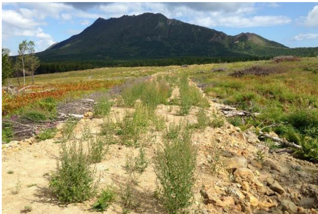
Photo 37 - Part of the cleared site for BS4
