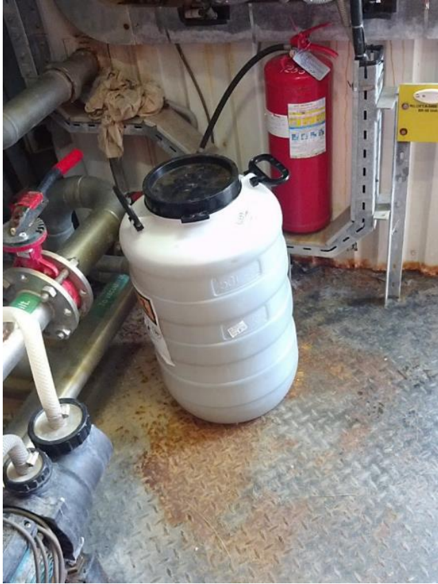
Photo 9 – Drum of polyaluminium chloride with no trip tray in the STP
