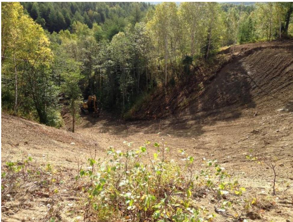
Photo 8 - KP 449 Restored slope in preparation of installation of ground anchors and netting
