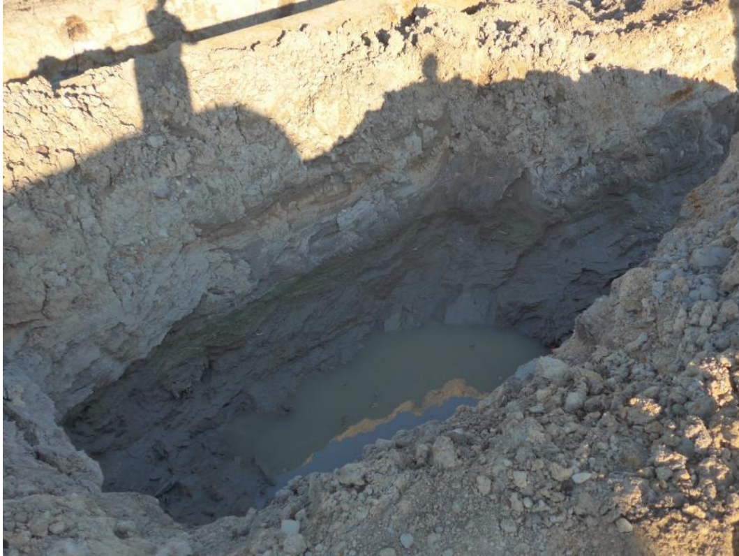
Photo 30 – Stormwater retention pit in the north of the OPF-C site
