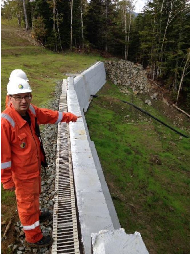
Photo 7 - Reinforced concrete retaining wall recently installed at KP 383.4
