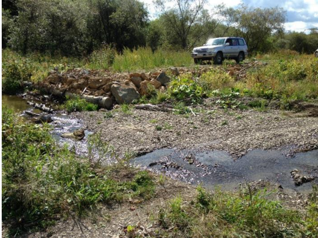
Photo 38 - Small watercourse crossing on access track to BS4
