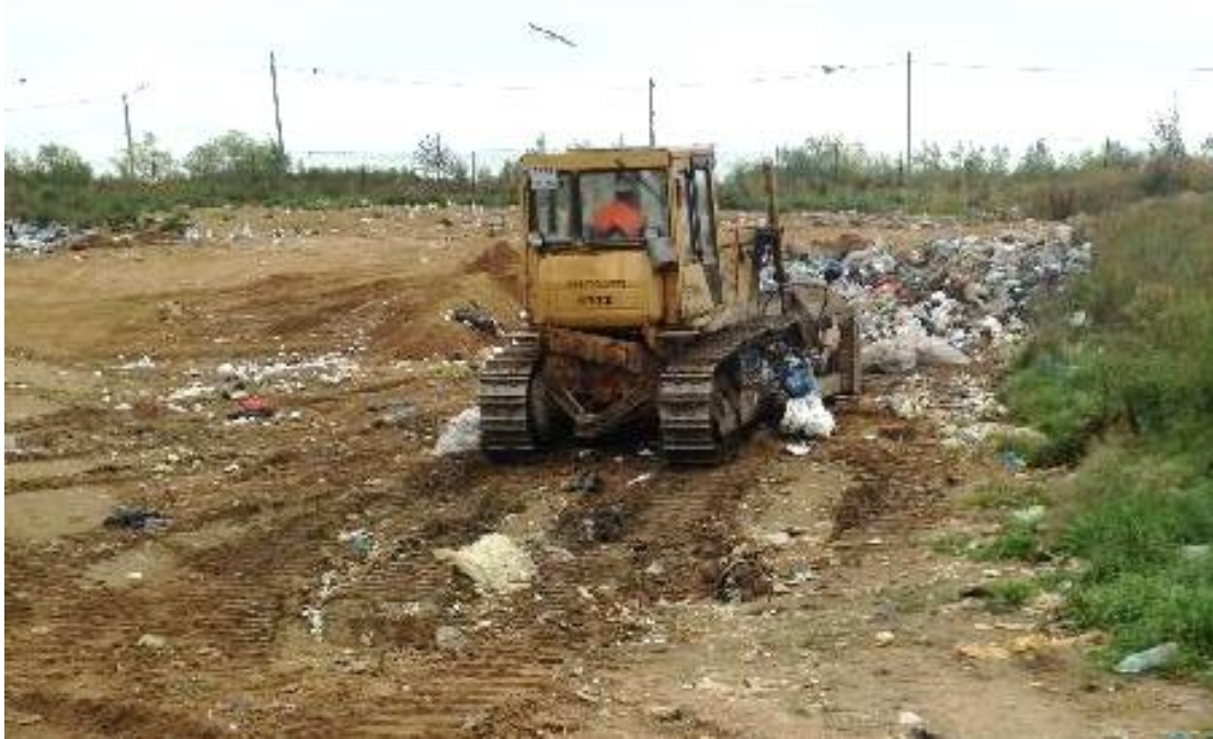
Photo 16 - Compaction and covering operations at Sakhalin Energy cell
