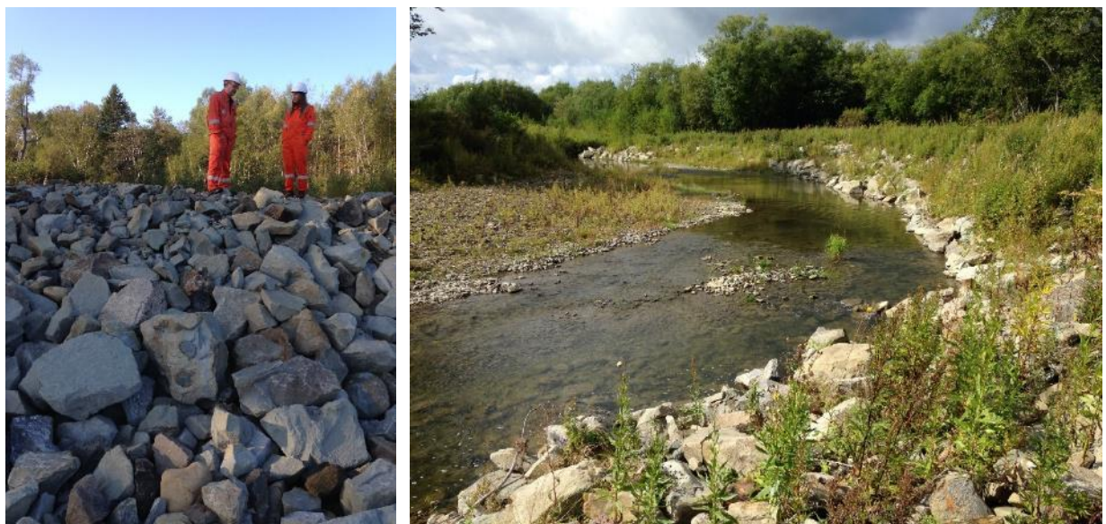
Photo 6 - Recently installed rip-rap, lacking vegetation (left)
