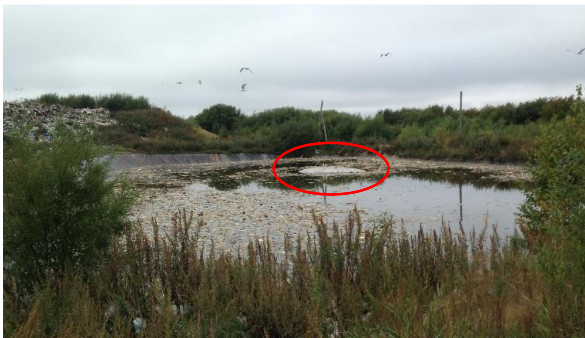
Photo 19 - Methane gas 'bubble' in centre of municipal cell leachate pond
