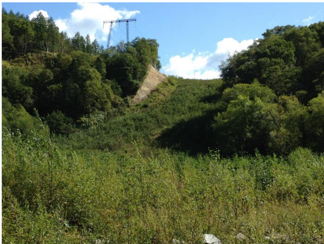
Photo 1 – En-route to KP499, steep slope on side of hill cutting
