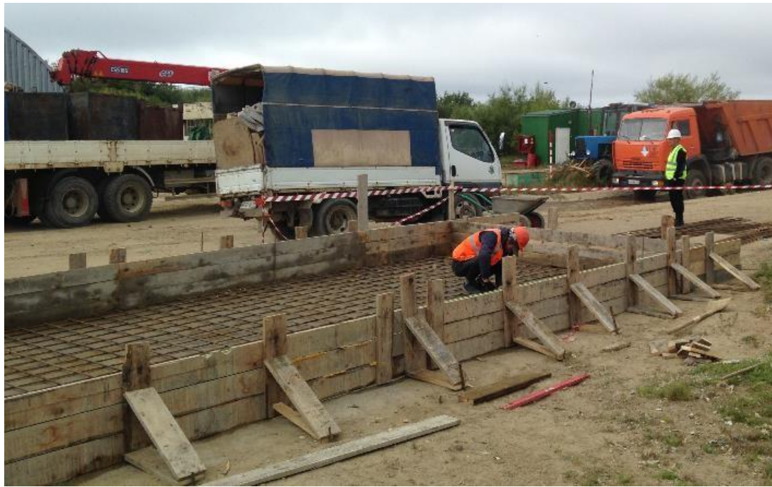
Photo 20 - New weighbridge under construction
