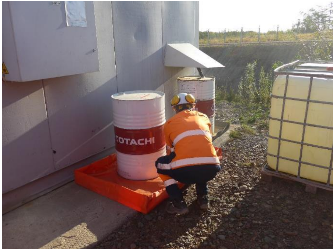
Photo 25 – Waste oil drum in a partially collapsed portable bund (it was being repaired when the photo was taken, after the auditor highlighted the issue)
