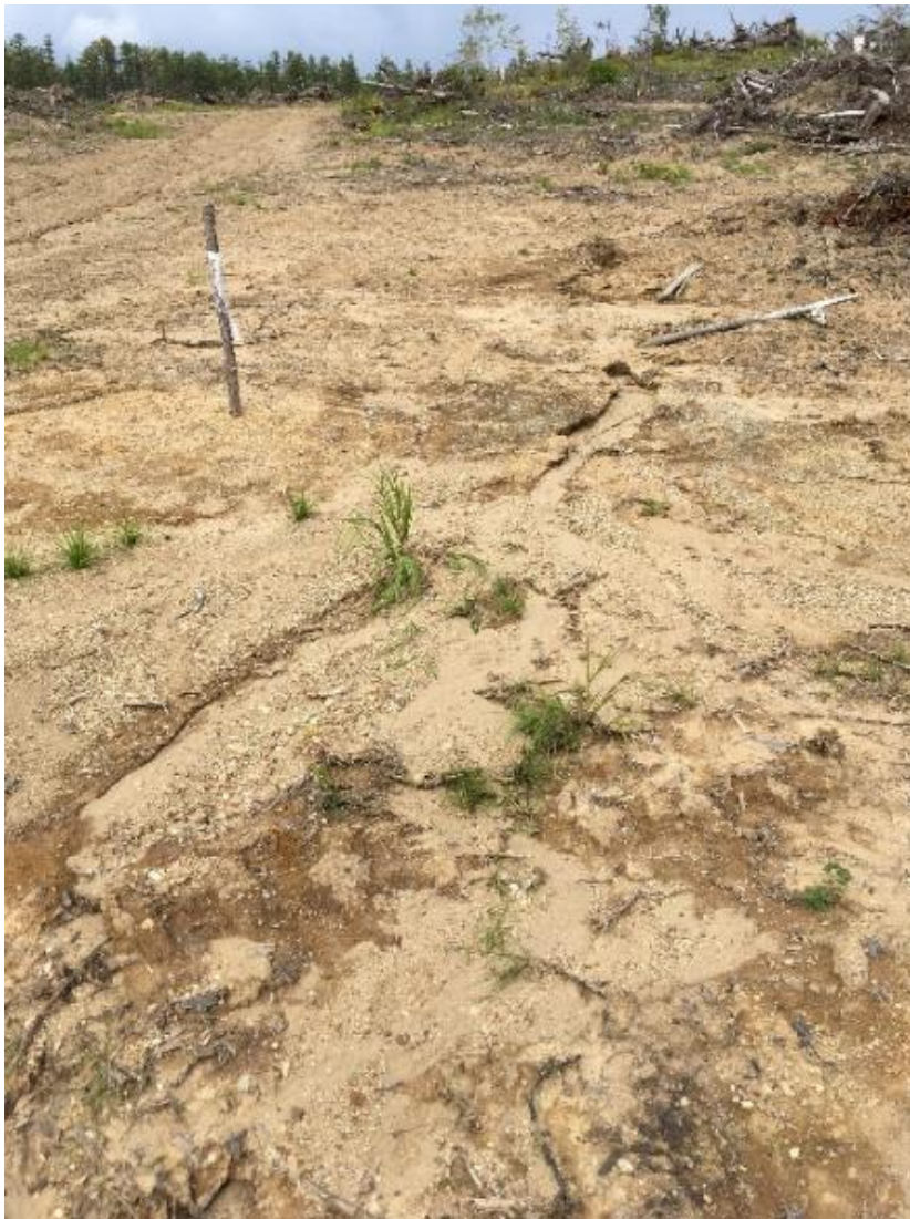
Photo 35 - Soil erosion within the proposed BS3 site
