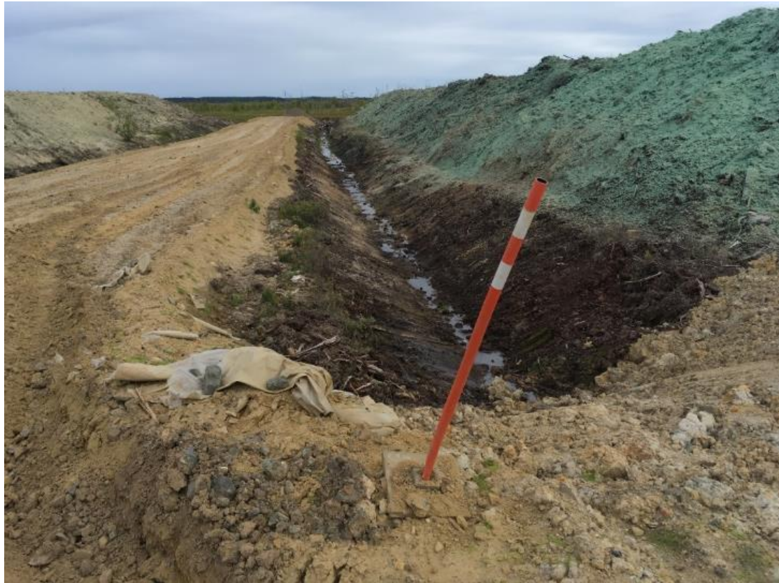
Photo 28 – Peat Storage Windrow and Adjacent Drainage Ditch
