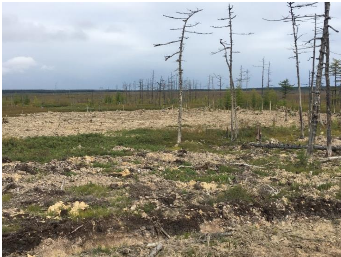
Photo 29 – Sub-soil that has been deposited beyond the active construction zone
